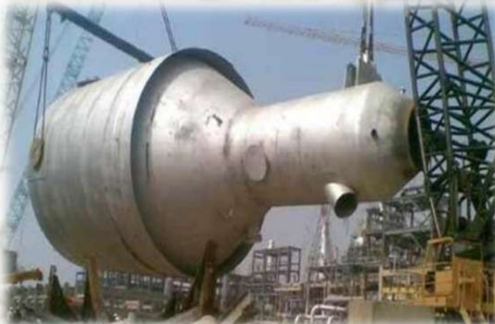
Reactor Under Erection
